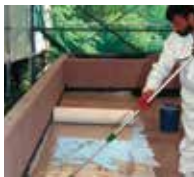
6. This is followed by the surface waterproofing ...
