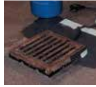
5. ... another generous layer of Triflex ProDetail is applied.
