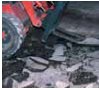
1. Old coverings are removed.
