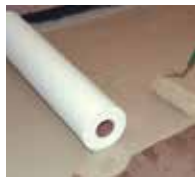
7. ... which is applied wet-on-wet with Triflex ProPark and Triflex Special Fleece.
