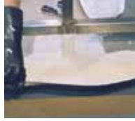
4. Triflex Special Fleece is applied across the entire surface ensuring there are no air bubbles.
