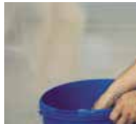
8. ... and dress with quartz sand in excess.
