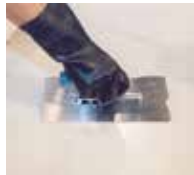
7. Spread the Triflex ProFloor coating using a trowel, level out ...
