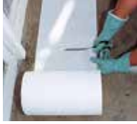
2. Prepare Triflex Special Fleece cut-outs.
