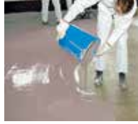
3. Spread the coating Triflex Than RG 568+ ...
