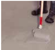
6. The surface is then finished with Triflex Pox Finish 173+.
