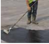
1. Prepare substrate, prime and dress surface.
