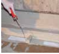
2. The details are waterproofed and fleece-reinforced with Triflex Than R 557 thix.
