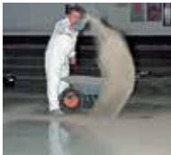
5. The wet coating is dressed with quartz sand.
