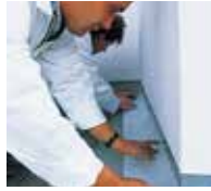
3. Insert Triflex Special Fleece, making sure that there are no air bubbles, and ...
