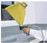
10. ... blow in Triflex Micro Chips.
