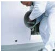
5. Spread the surface coating Triflex ProFloor ...
