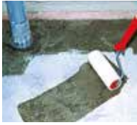
1. Prime wall junction and surface.
