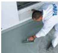
6. ... using a trowel, and ...
