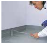
8. First apply the finish Triflex Cryl Finish 205 to the details, ...
