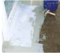
4. Apply Triflex Special Fleece across the entire surface, removing any air bubbles.
