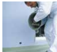
10. The wearing surface: Spread and level out Triflex ProFloor ...
