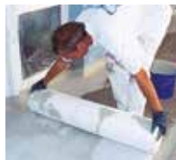
8. Triflex Special Fleece is applied across the entire surface, removing any air bubbles.
