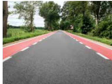
K40, Halle / Getelo (DE) • Project: Cycle lane marking • Project size: 7.0 km • Systems: Triflex Precryo Line 300, Triflex Precryo Cryl Cold Plastic 2K
