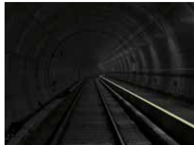
Underground, Hamburg (DE) • Project: Underground tunnel U4 • Project size: 5.6 km • System: Triflex Precryo Line 300 NightLine
