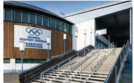
Olympia Ice Sports Stadium in Garmisch-Partenkirchen (Germany)
